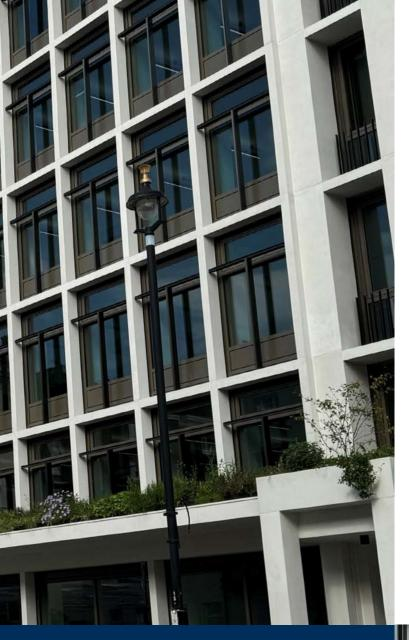
"The largest units spanned 11 metres and weighed more than 15 tonnes. Each piece was finished with a combination of etched and polished surfaces to achieve the required aesthetic quality and durability."
