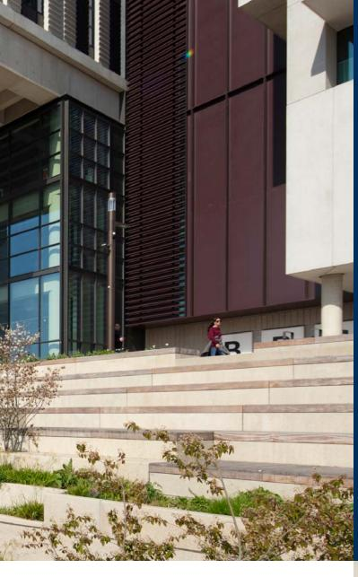
"Over 700 bespoke precast units were manufactured, including terraces, stairs, landings, walls, benches, planters and paving."
