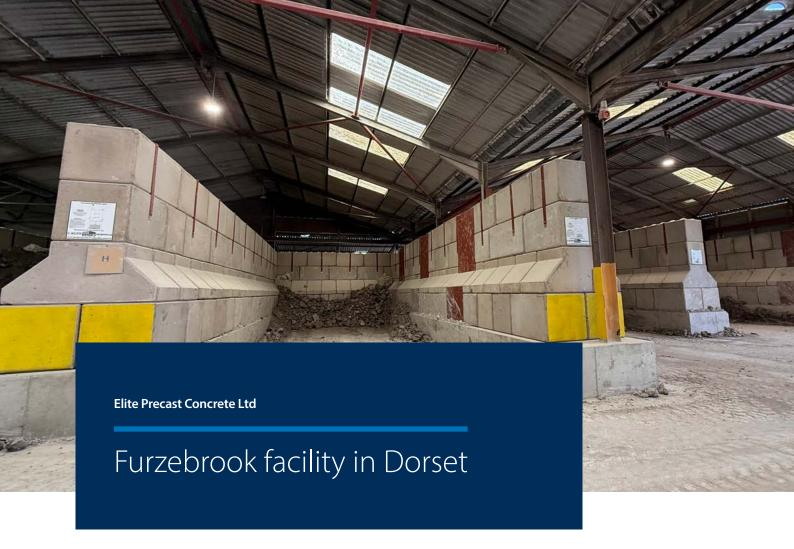
IMERYS, a mineral-based speciality solutions company, has recently completed a major refurbishment of its Furzebrook facility in Dorset. The works addressed the replacement of ageing steel columns and wooden sleeper walls, which had deteriorated over time, causing structural failures. These failures were limiting storage capacity and allowing cross-contamination between different grades of stored materials, undermining product quality, profitability and overall operational standards.
