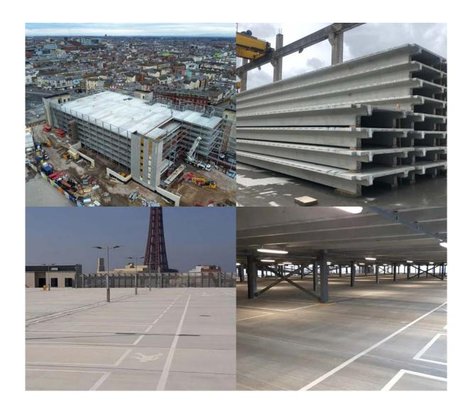
"The design of these units was carefully engineered to ensure they met a minimum 3.5 Hz natural frequency for vibration control, all while maintaining a lightweight profile."
