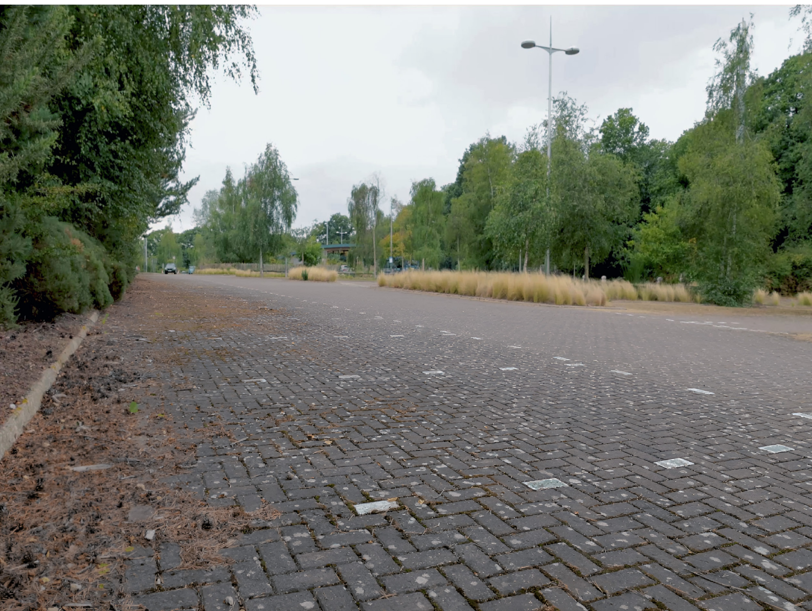
17 years after construction there are no issues resulting from tree roots in the CBPP sub-base.
