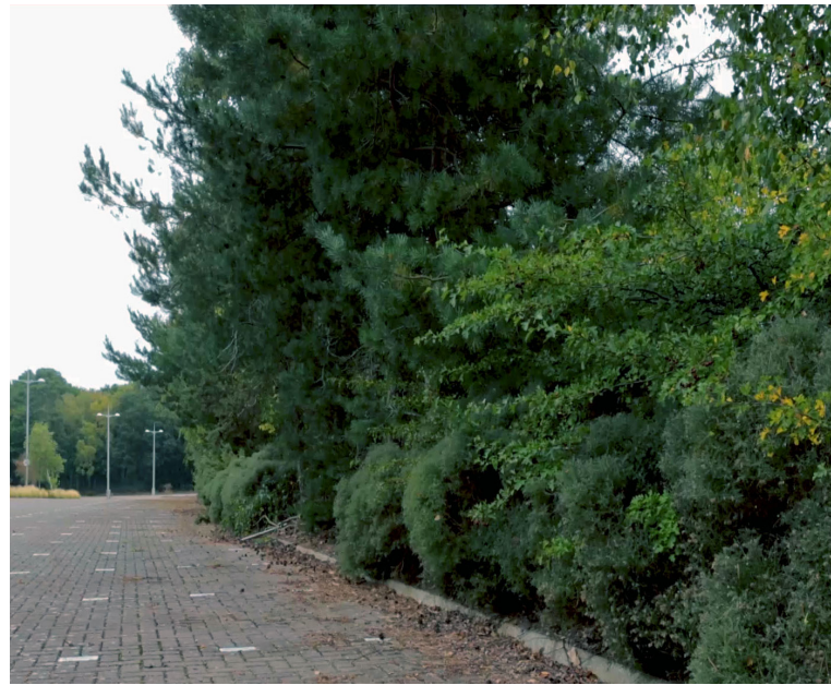
17 years after construction there are no issues resulting from tree roots in the CBPP sub-base.
