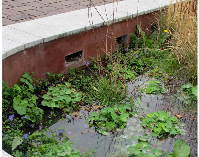
The original road surface has been replaced with attractive, 'self-draining' concrete block permeable paving. Clean water from the permeable paving passes into the planted basins. The 'wiggly wall' feature meanders through both paving and planting.
