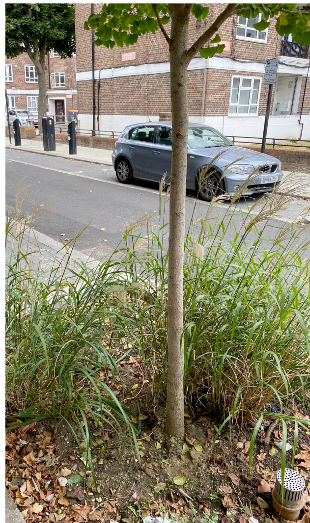
Excess water is discharged from the raingardens to the sewer via infiltration and overflow pipes
