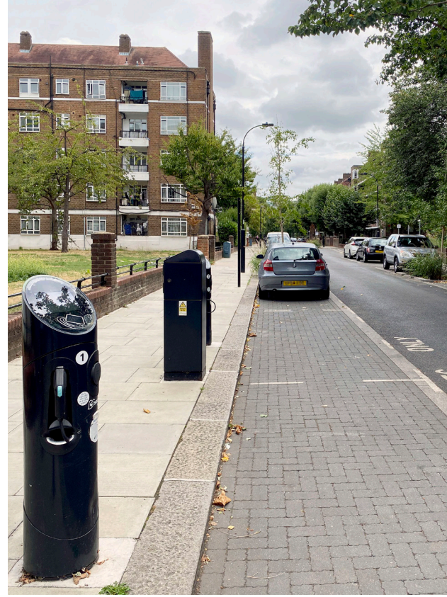
Permeable paving parking bays include provision for electric vehicle charging
