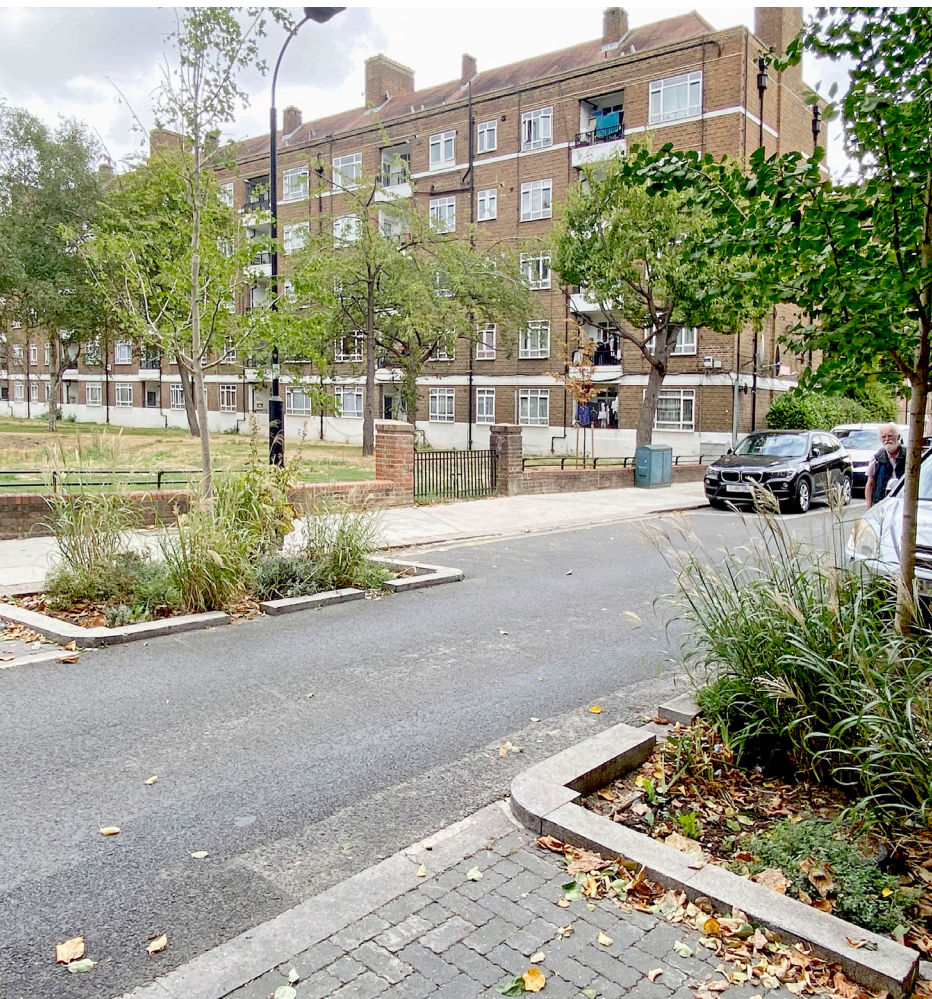
Raingardens between permeable paving areas incorporate new tree planting with long-term, passive sustenance
