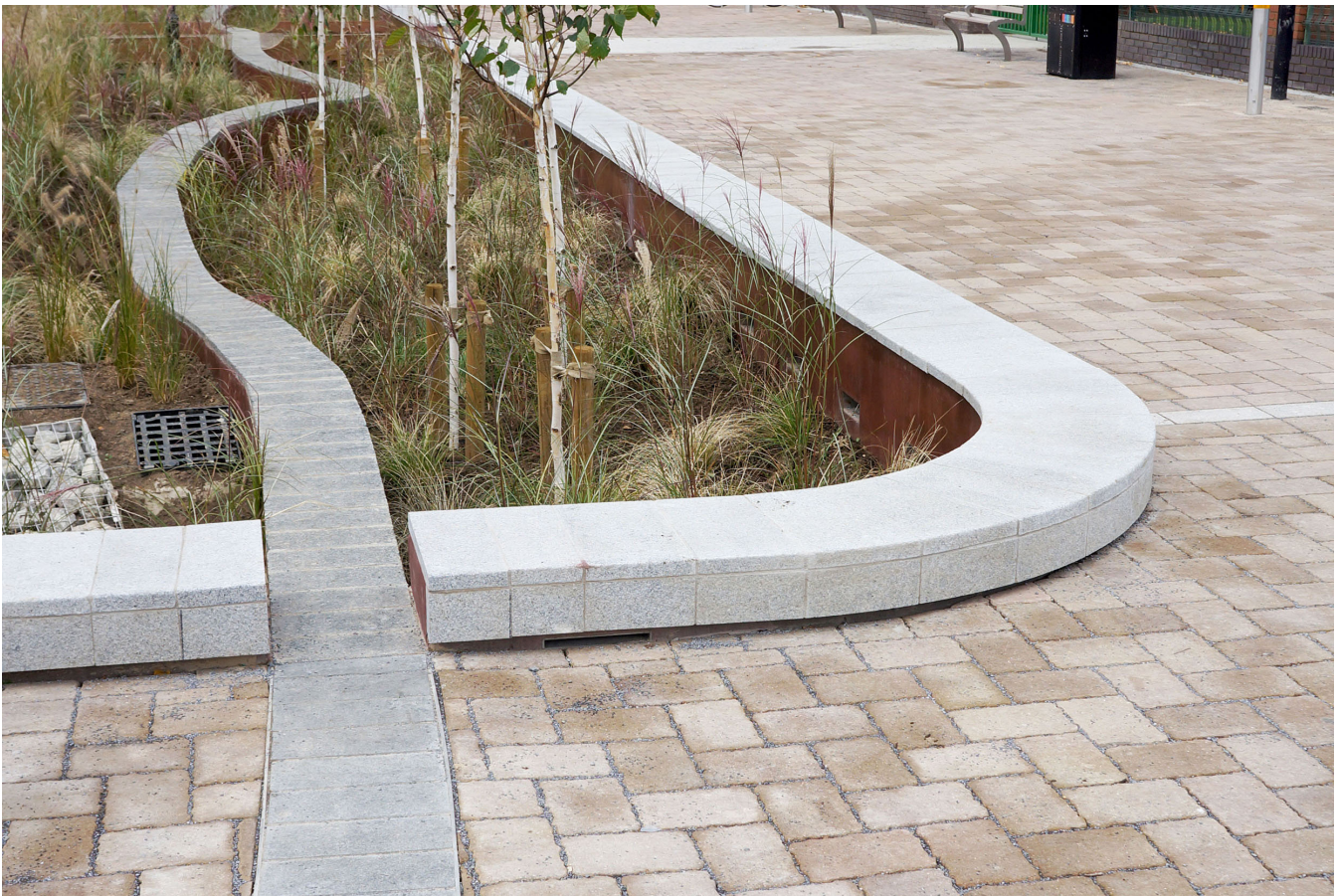
The original road surface has been replaced with attractive, 'self-draining' concrete block permeable paving. Clean water from the permeable paving passes into the planted basins. The 'wiggly wall' feature meanders through both paving and planting.
