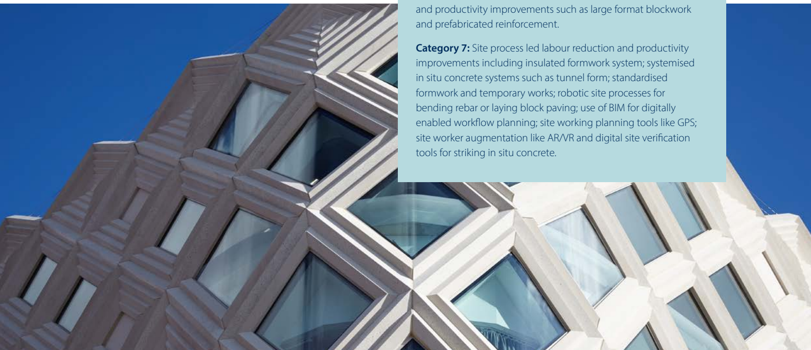
The facade of Victoria Gate in Leeds combines polished and acid-etched precast concrete finishes in a tour-de-force of geometry and texture. Architect: ACME; Structural engineer: Waterman Group; Precast concrete cladding: Techrete. Image courtesy of British Precast.
