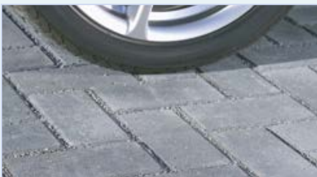
Permeable paving should have permeable aggregate filling the joints
