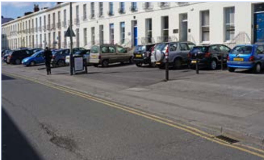
Off-street parking and drives draining onto the road add to public drainage loads and should be addressed.
