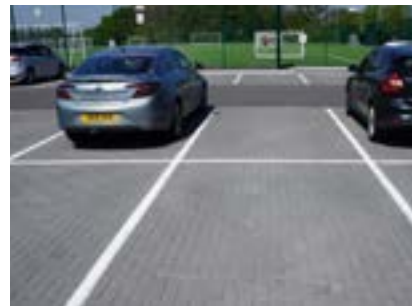
Rainwater from impermeable asphalt is collected by concrete block permeable paving and stored in permeable sub-base beneath both surfaces.
