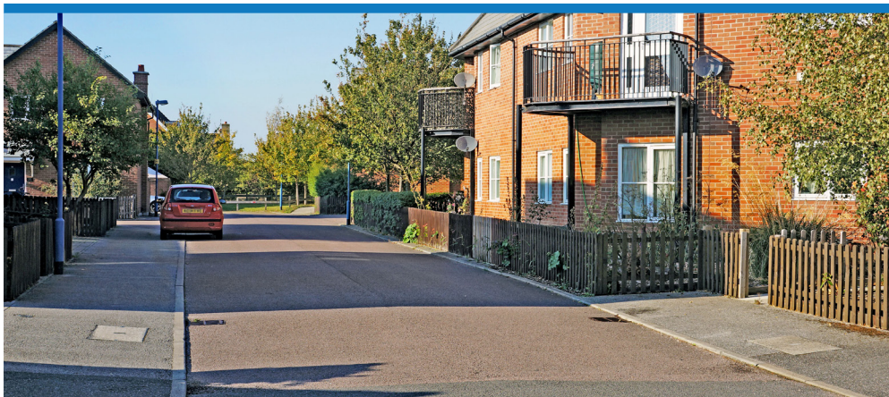
The access road is characterised by continuous asphalt surfaces, served by numerous road gulleys discharging directly to piped drainage.
