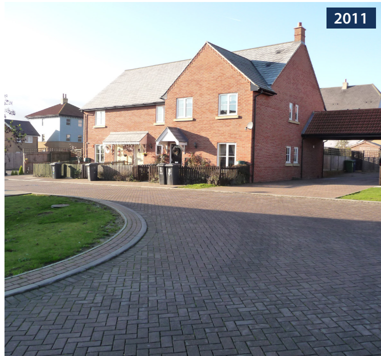
Concrete block permeable paved carriageway in Catchment A, accepting runoff from conventional block paved drives and parking areas. Concrete kerbs laid flat delineate road edges.
