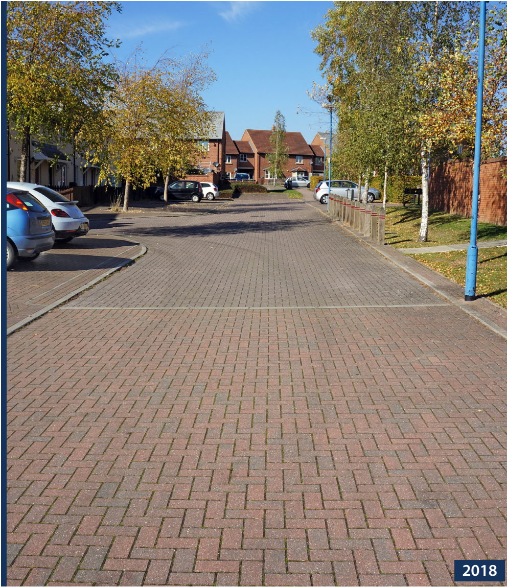
Conventional block paved road, driveways and parking areas in Catchment B all drain onto the permeable paved central carriageway.
