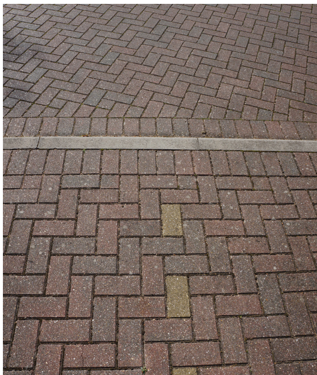
Concrete block permeable paving some 13 years after completion.
