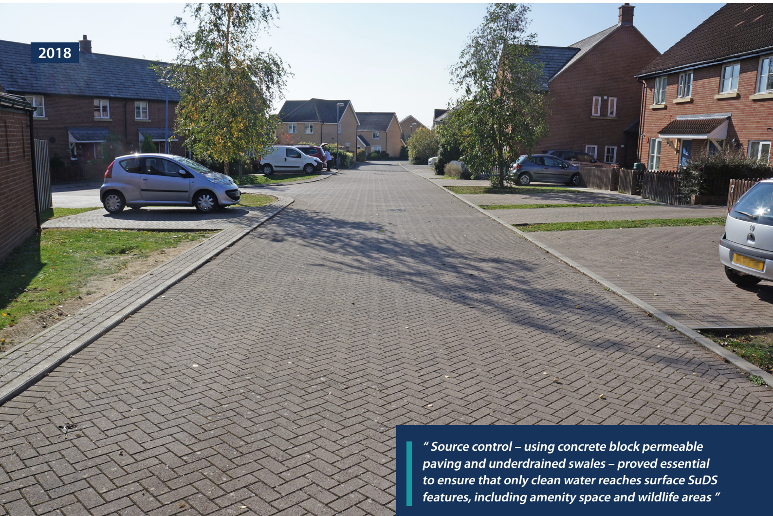
Concrete block permeable paved carriageway in Catchment A, accepting runoff from conventional block paved drives and parking areas. Concrete kerbs laid flat delineate road edges.
