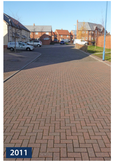
Conventional block paved road, driveways and parking areas in Catchment B all drain onto the permeable paved central carriageway.
